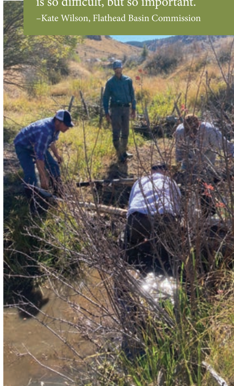
Members of the Idaho Rangeland Conservation Partnership steering committee worked with ranchers and the Idaho Department of Fish and Game to build beaver dam analogs that will help with stream restoration on the Josephine Ranch.
